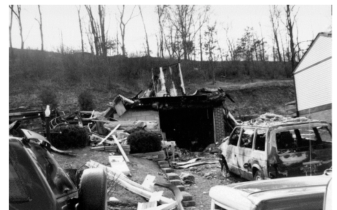
Figure 2. Photograph of a house in western Pennsylvania that exploded and burned as a result of natural gas leaking into the basement from a nearby gas well. The gas built up in the cellar and ignited when the furnace fired up. Photo courtesy of Fred Baldassare
